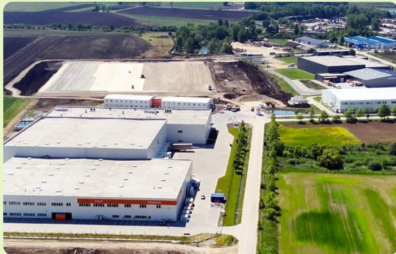
Intretech Hungary Kft. also jointly built the first overseas solar-storage-charging smart power station with Shanghai Sunnic new energy technology Co., Ltd. This project marks an important milestone in the company's layout in the European new energy market.
